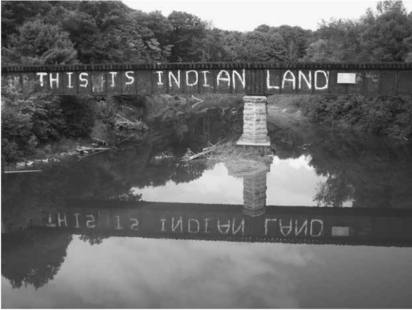
Image 2: Rail bridge spanning the Garden River. Photo: Karl S. Hele.
